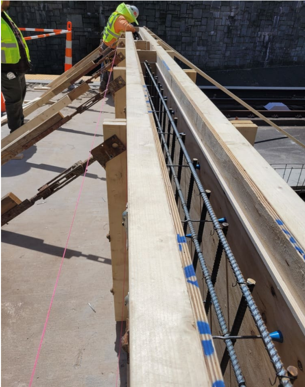
Installing end walls on renovated platform
