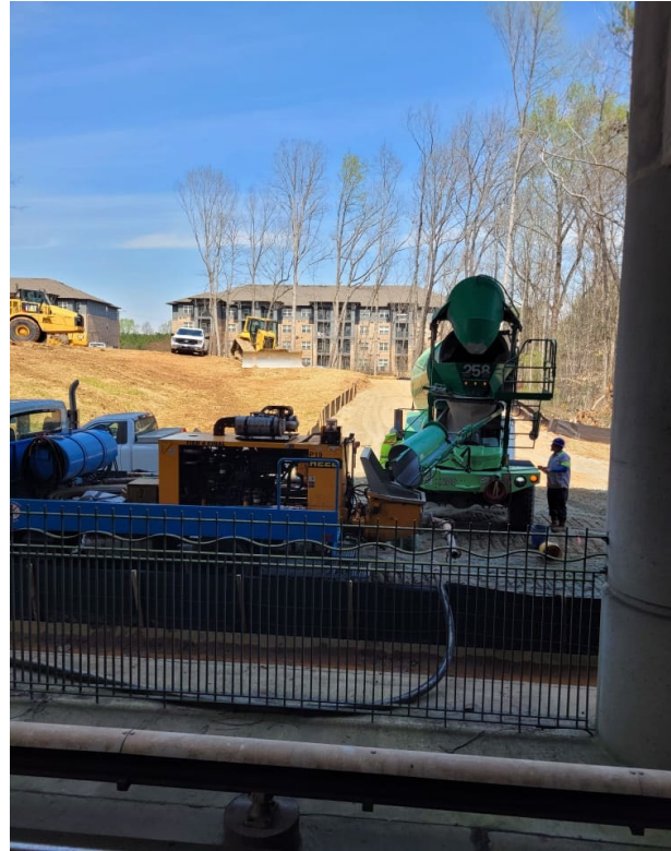
Concrete pouring for new platform
